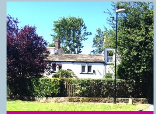
Hederows, verges, trees and walls all contribute to the conservation area
