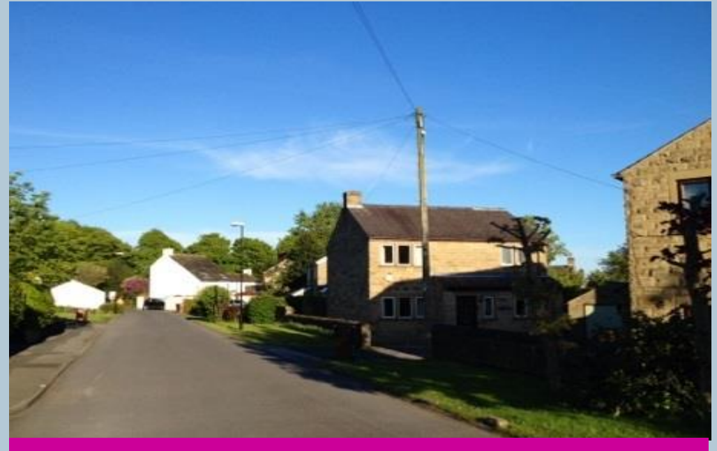
Burnt Side Road; the mix of old and new houses together with trees and green spaces adds greatly to the character of the Conservation Area.
