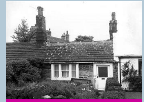
Historic Photograph: single storey cottages on Moor Top (1700s -1800s) are a rare survivals of this type in West Yorkshire.
