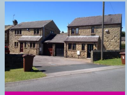
New stone housing development on Burnt Side Road.
