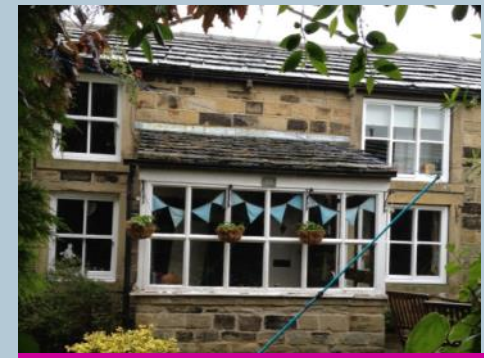
5 and 6 Moor Top, late 18th century, Grade II listed. Originally two cottages now one.
